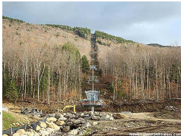
The Lincoln Express Quad under construction on South Peak (2007)
